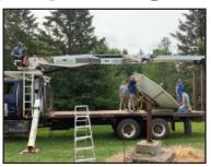
new, more stable pedestals are immune to the frost heave and new cable and hardware were also added to the project to ensure the highest possible signal quality.
